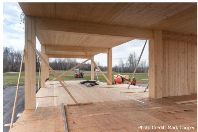
Cross-Laminated Timber, Glulam and Dowel-Laminated Timber are some of the mass timber products used in the structure.
