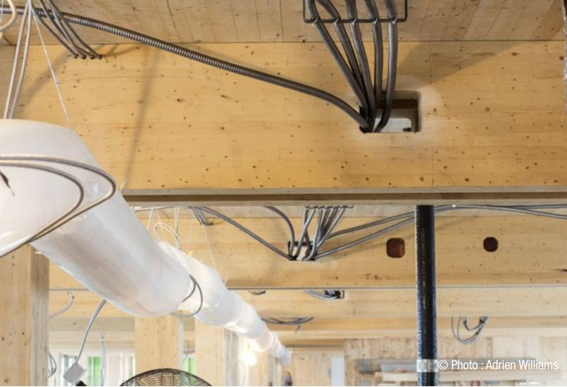
Beams with pre-drilled holes for machinery
