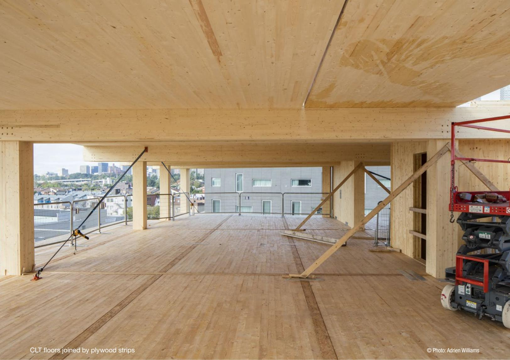
CLT floors joined by plywood strips
