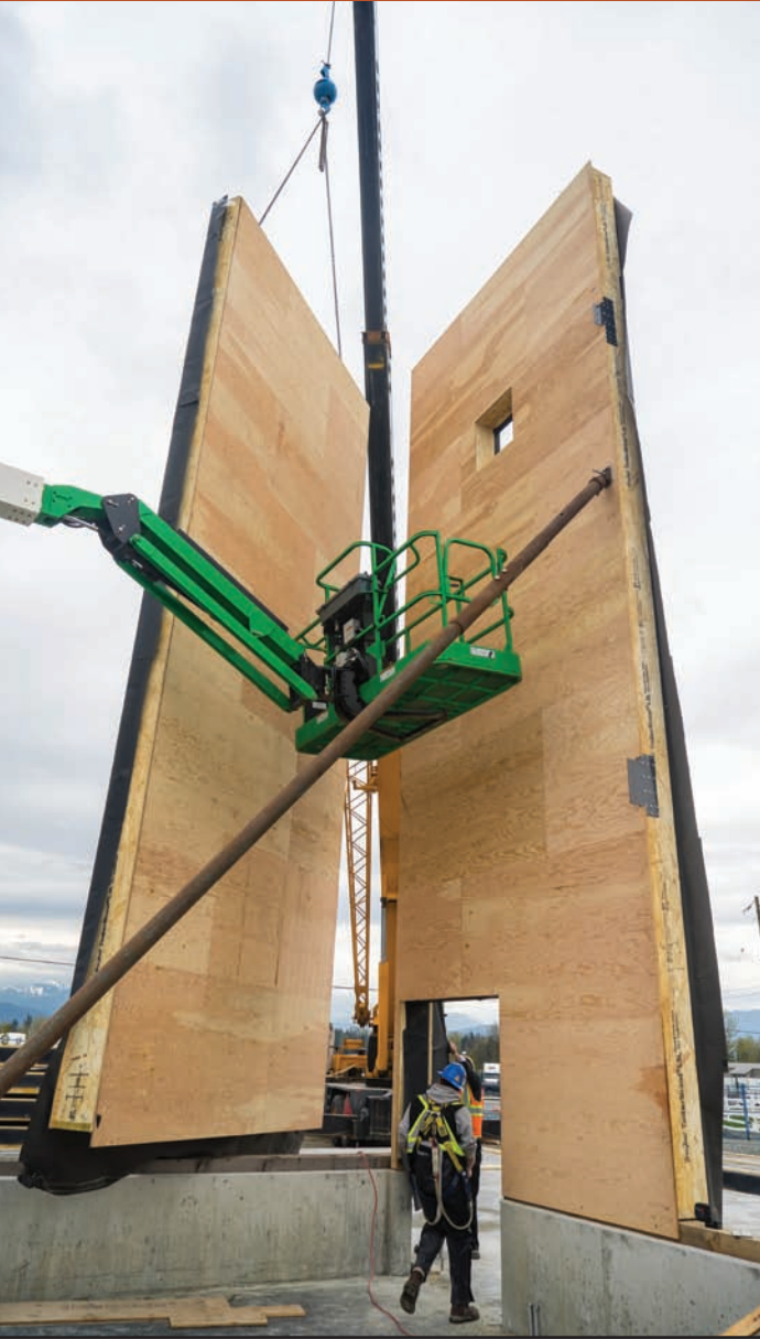
Fig. 4.5: Wall panel being placed
