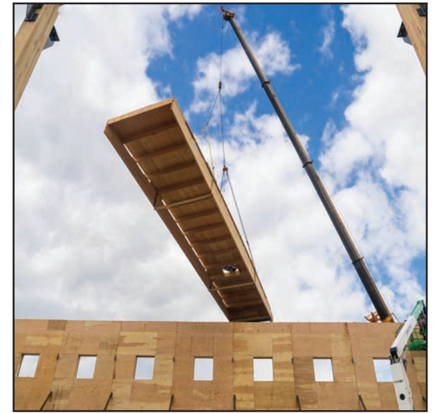
Fig. 4.4: Roof panel being lifted into place
