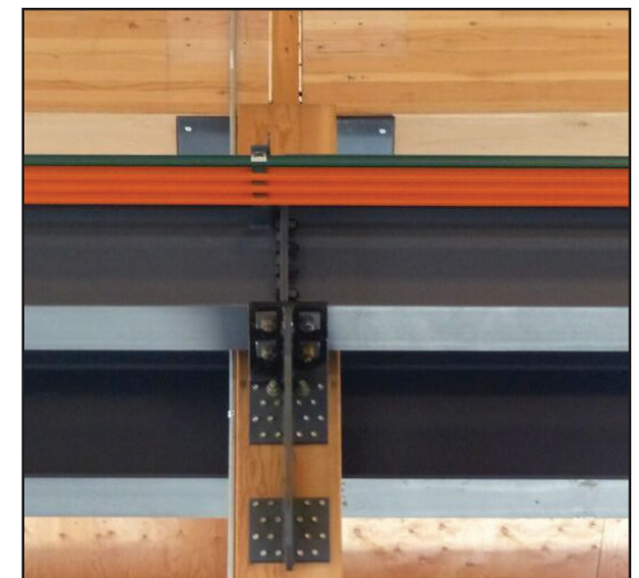
Fig. 4.11: Column-to-beam connection at gantry crane
