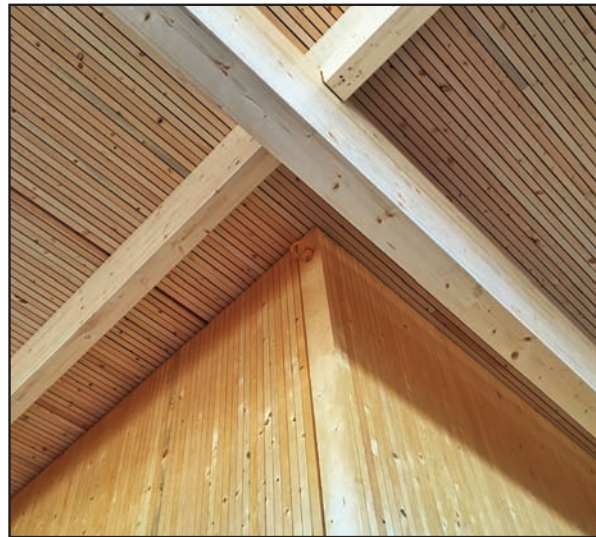
Fig. 4.14: DLT panels in the office area
