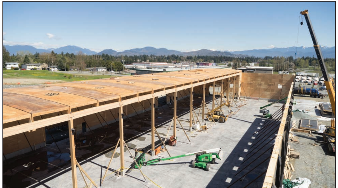
Fig. 4.10: The cambered roof beams create a sloping roof surface that facilitates drainage
