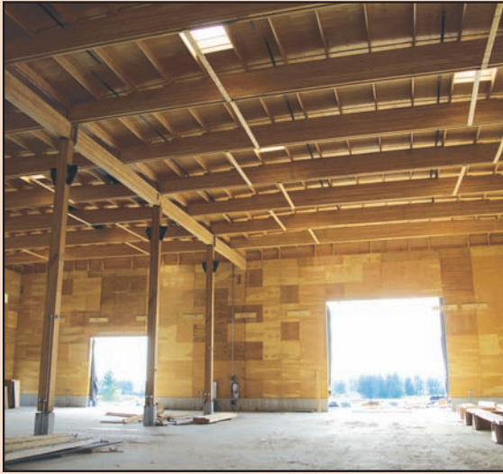
Fig. 4.9: The end walls with openings were designed as coupled shear walls, eliminating the need to provide cross-bracing for lateral resistance
