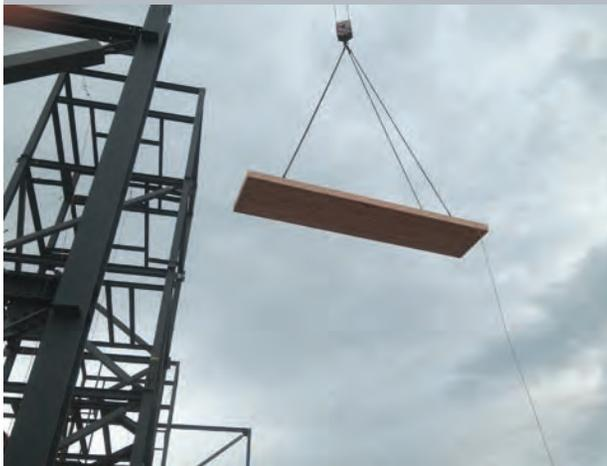
Floor panels were lifted into place by crane
