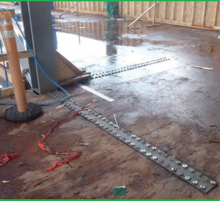
Steel strap tying wood floor to steel frame for lateral bracing
