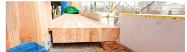
A section of the perimeter beam that resists the horizontal forces on the external wall of the building
