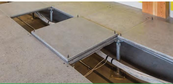
Access flooring. For a building of this size and type, the concealed space must be non-combustible.
