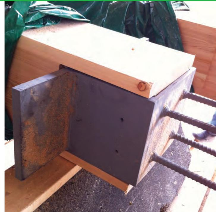
The columns have end-to-end bearing to minimize shrinkage over the height of the structure. Rebar rods on the saddle connector fit into holes drilled in the base of the column above.
