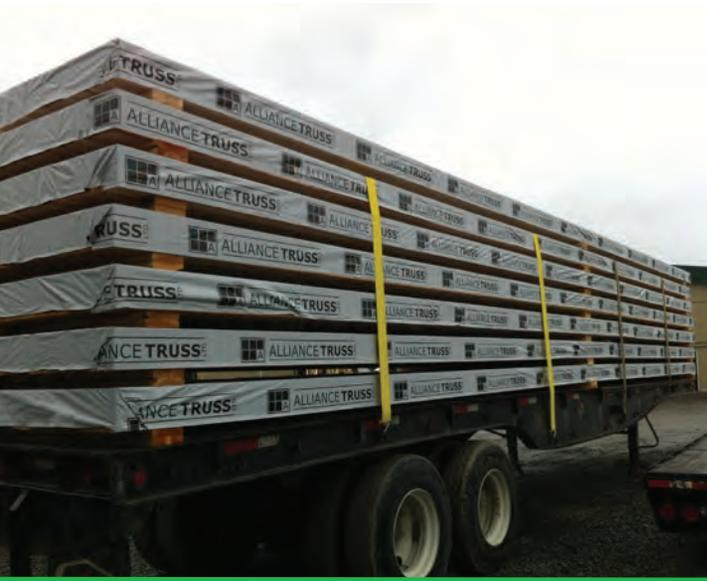
Prefabricated floor panels are delivered to site for installation
