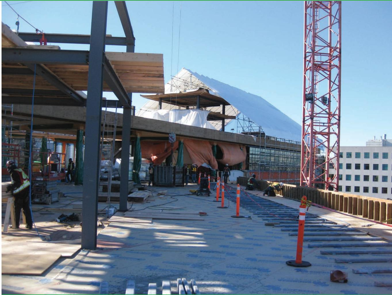
A tent was erected to protect the wood structure from inclement weather during erection and prior to closing in
