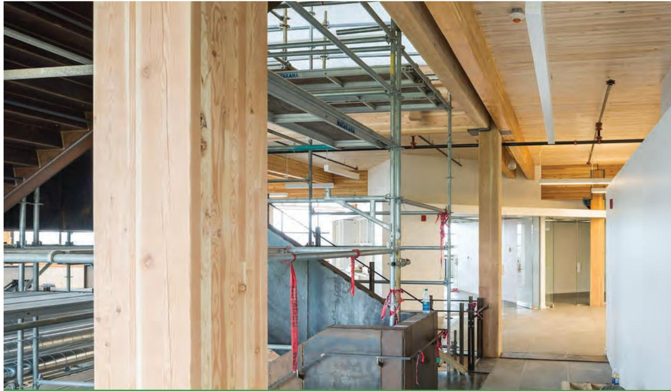
The dropped beams around the perimeter of the atrium are designed to contain smoke in the case of a fire
