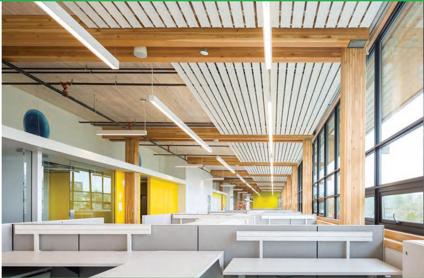
Radiant ceiling panels are positioned alongside the windows to provide additional heating or cooling as required
