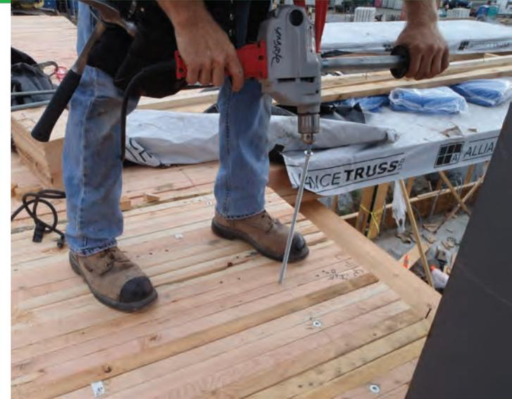
Once in place, the floor panels were lag screwed into the glulam beams
