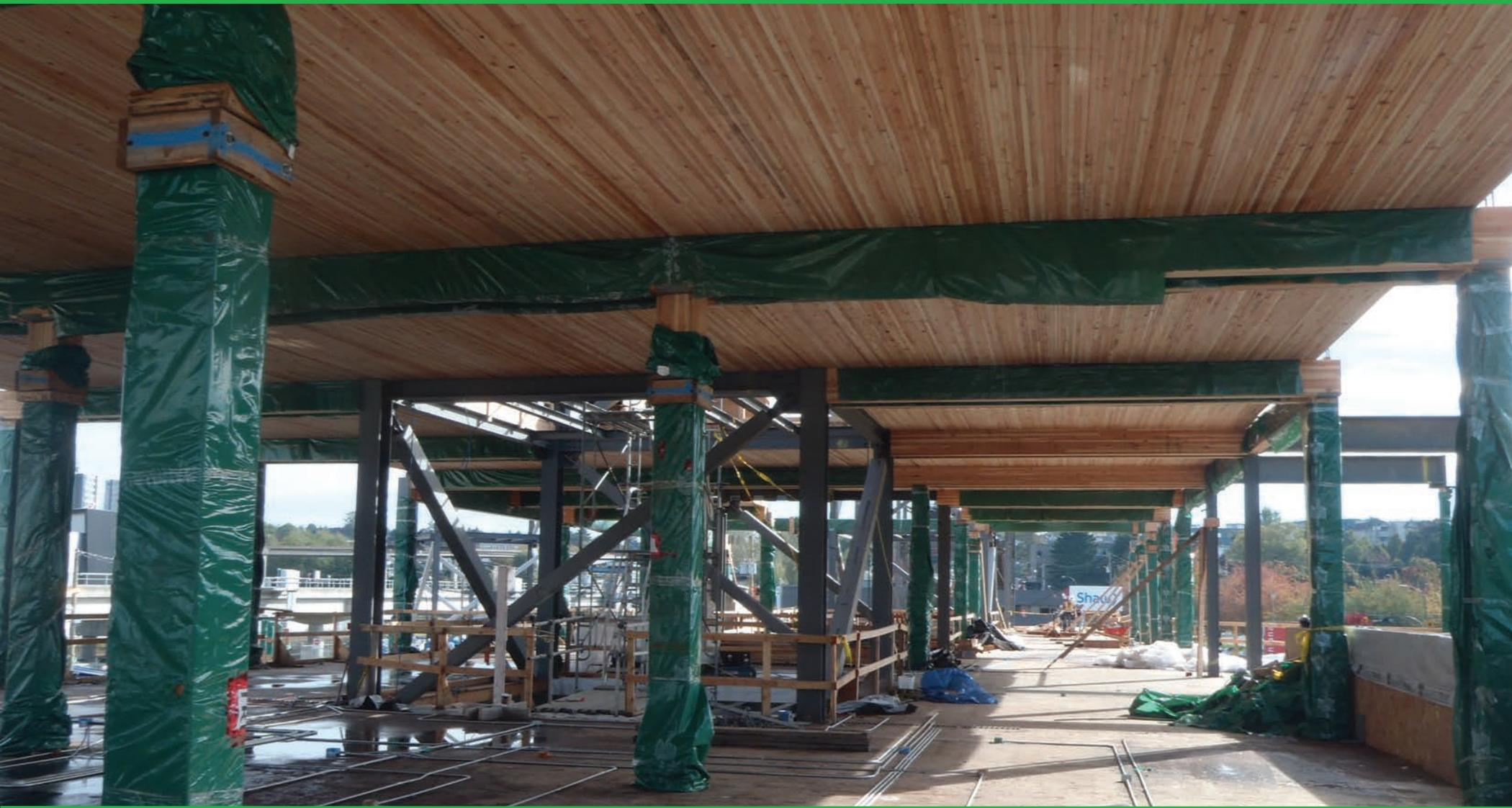
The nail-laminated floors are tied into braced steel frames that provide lateral resistance to the structure
